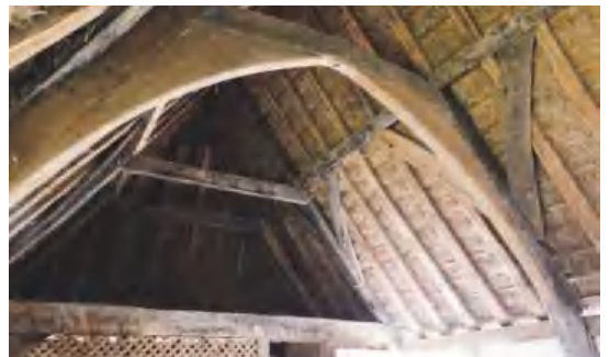
The interior showing the crucks supporting the roof timbers Photograph courtesy of G. Grime, Weald & Downland Museum
